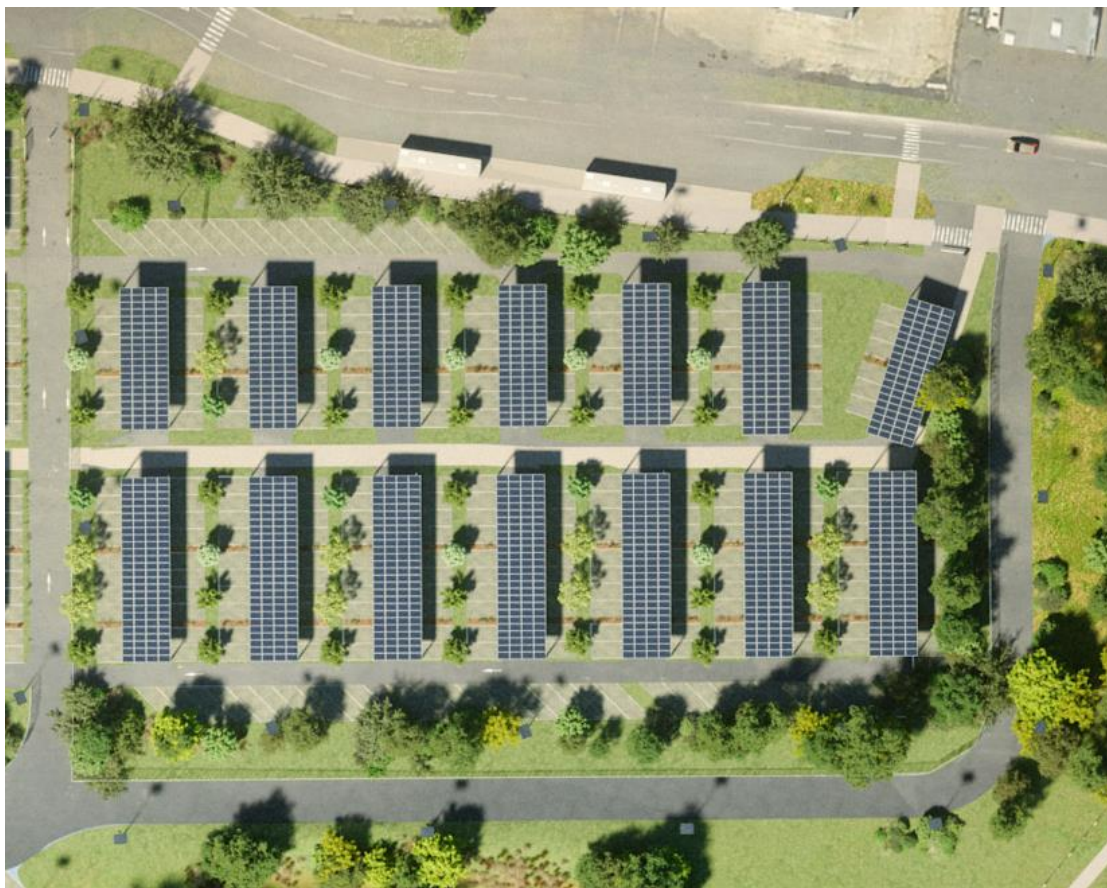
Figure 6 : Parking public – source François de la Serre
